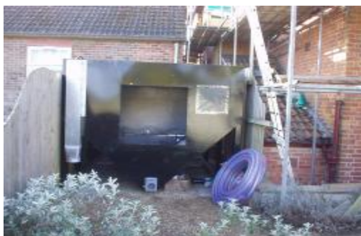
Purpose built bulk hopper
