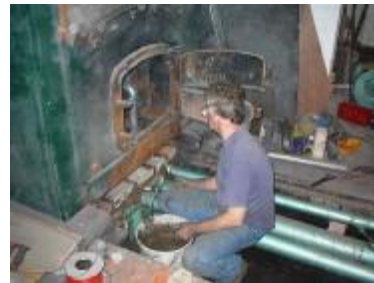
Replacing the under stokers
