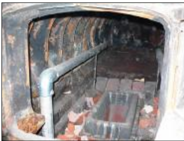
Secondary air in boiler
