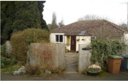
Boiler and store in adjacent outhouse
